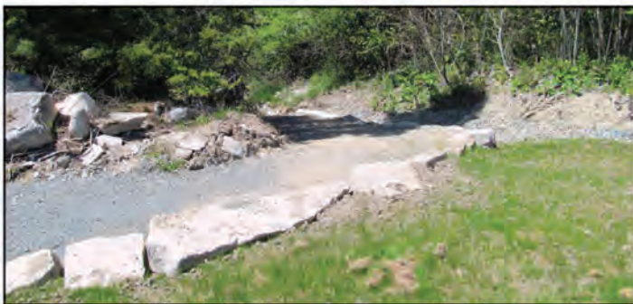
Photo by Lisa Herrington New ramp at Gordon's Wharf.
